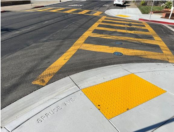
Multiple high visibility crosswalks and ADA curb ramps were installed on Spruce Ave. and Lux Ave.
