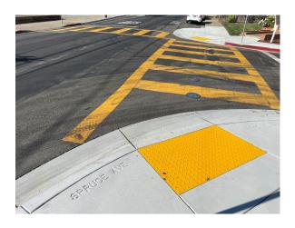
Multiple high visibility crosswalks and ADA curb ramps were installed on Spruce Ave. and Lux Ave.
