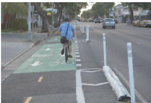
The bike lane can be painted with buffered (wide) lane lines and physical separators on both sides, separating them from the drop-off curb lane on the rider’s right, and the downhill travel lane on the rider’s left. The photo at left illustrates how curbing material and flexible, reflective delineators can separate bicycle and travel lanes.
