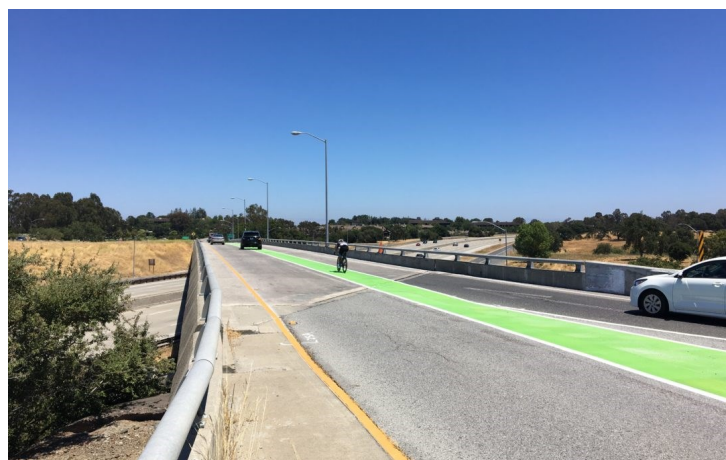
Photo: SVBC, Sand Hill Road Overcrossing
