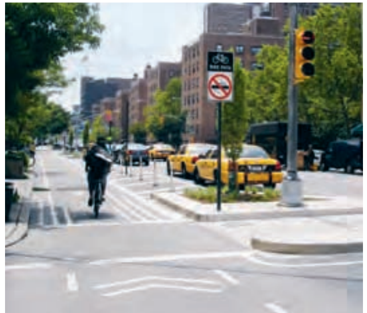
Physically separating bicycle from vehicular lanes along busy roads creates more comfortable and convenient bicycling environments.
